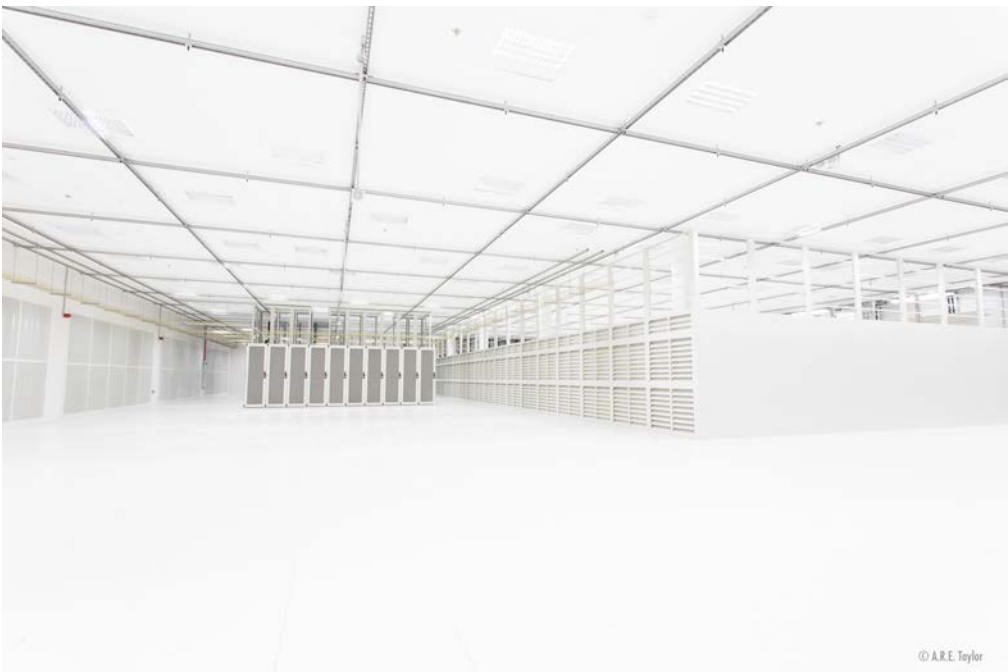
Figure 5: Servers wait on standby in a cloud provider’s back-up data centre. Photo by A.R.E. Taylor.
