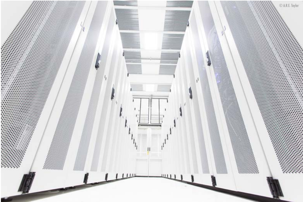
Figure 4: Cloud data is stored on the hard drives of servers (pizza-box shaped computing machines), which are securely encaged inside cabinets arranged in aisles. Photo by A.R.E. Taylor.
